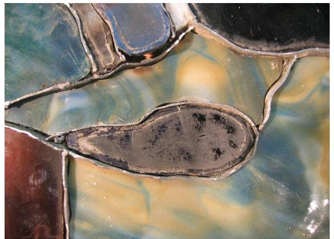
Each piece of glass of the first layer removed is then laid on a glass tray in its exact location on the panel.
