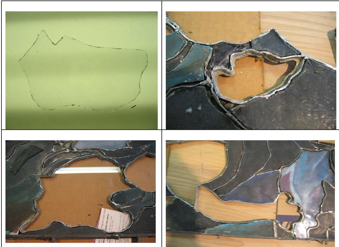
When all the leads have been peeled and that the pieces of the first layer have been removed and laid apart on a glass tray, the second layer is also removed and laid on another tray. The naked structure of the leads appears very clearly.
