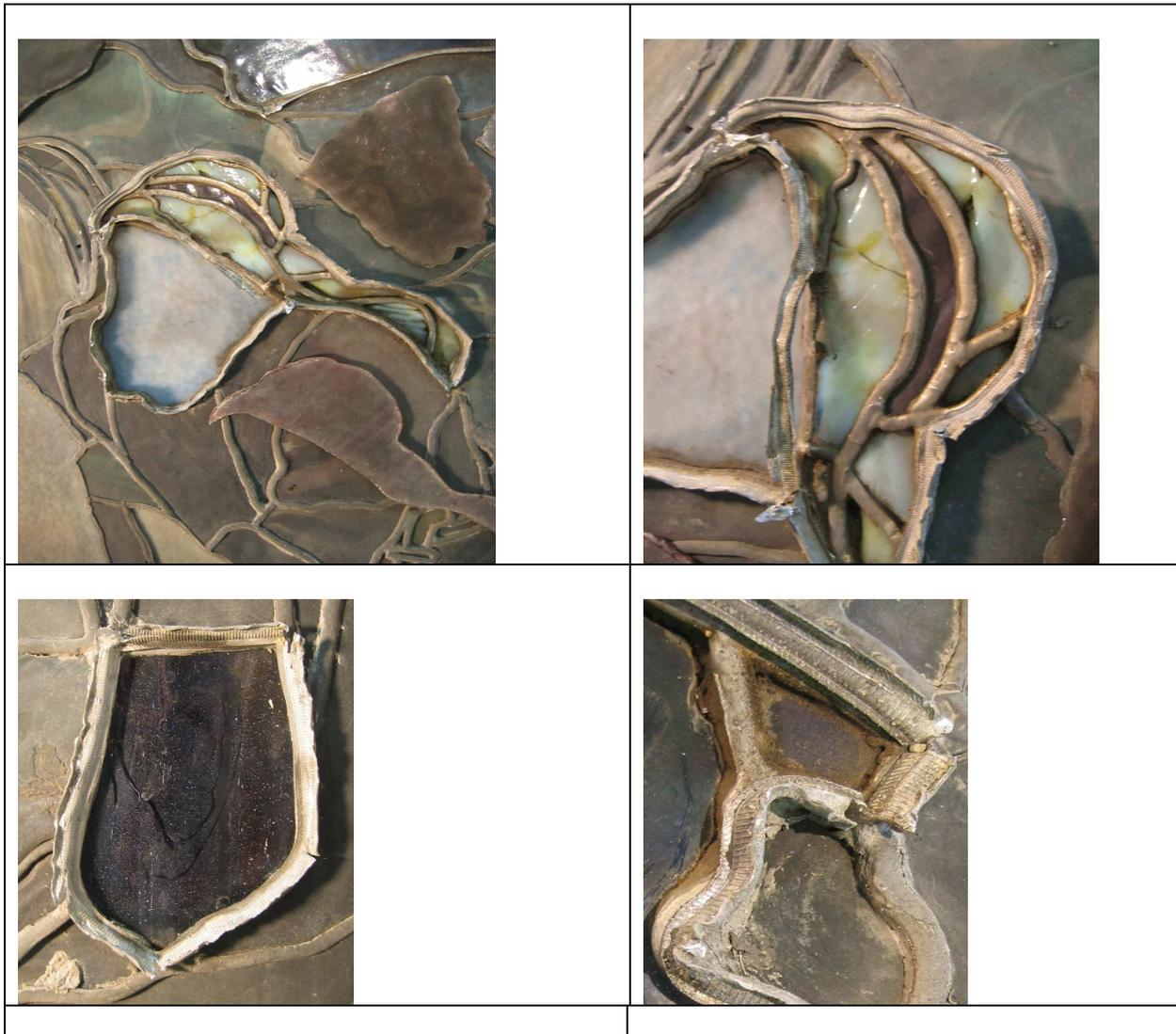
The wings of the leads have been lifted up to remove the plated piece of glass.
